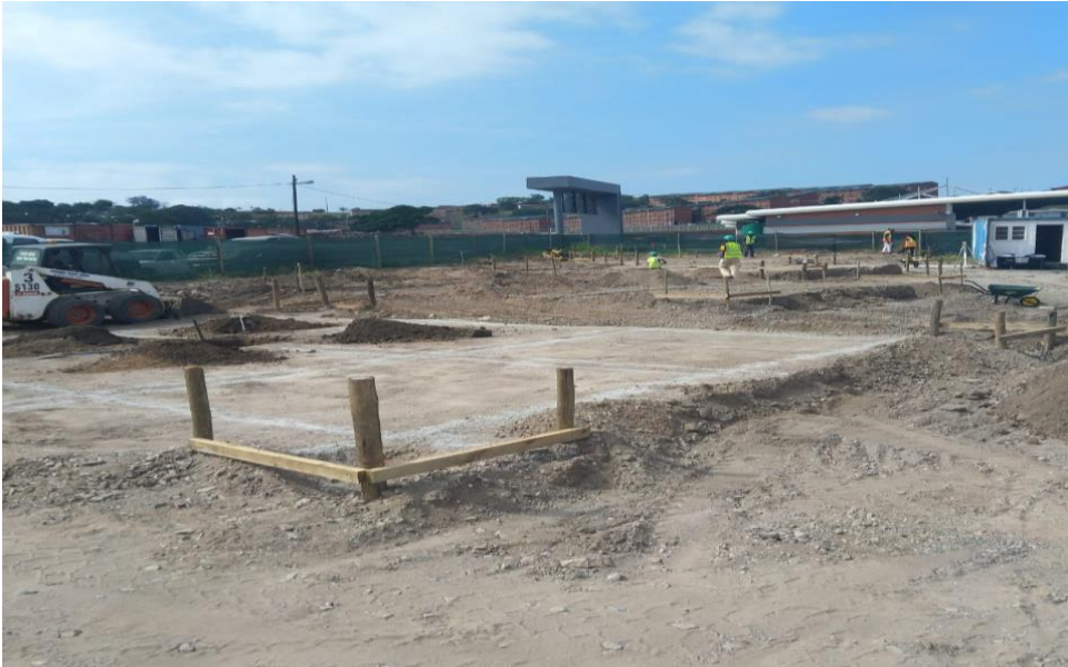
Ezimbuzini Informa Traders Stalls (Phase 2) – at Sub-Structure level – R19 000 000.
