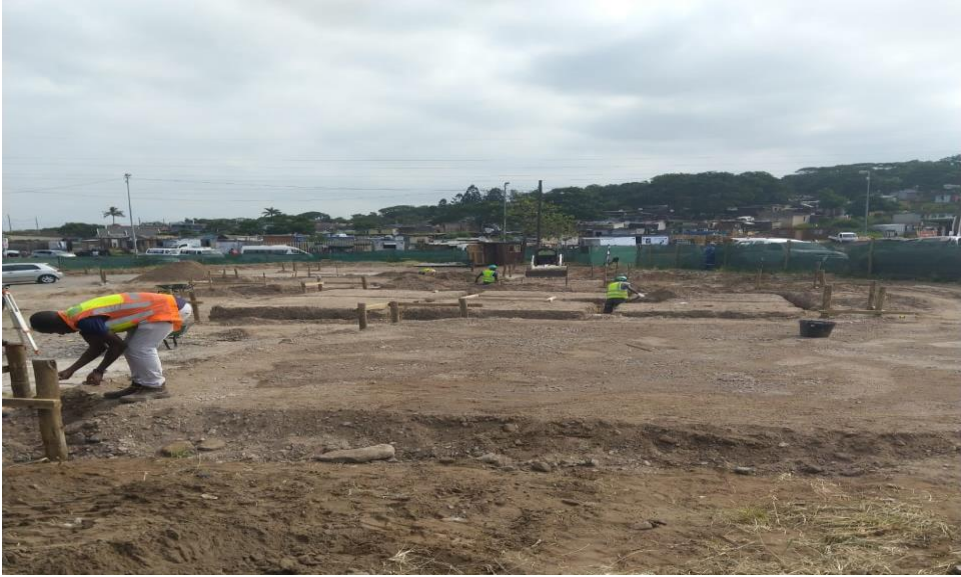
Ezimbuzini Informal Traders Stalls (Phase 2) – at Sub-Structure level – R19 000 000.00
